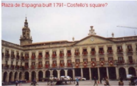
Plaza de España built 1791, Costello's square?
